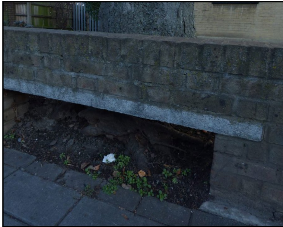
Photograph 4 – Example of wall bridge over tree roots
